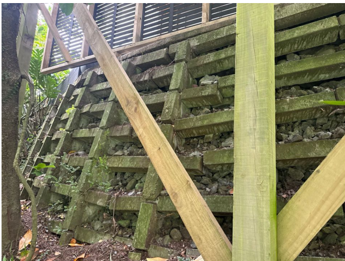
The concrete crib retaining wall is solid and secure
