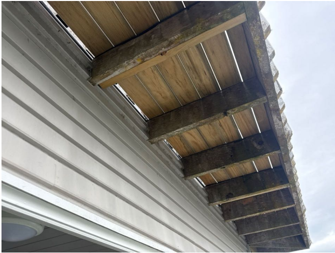
The cantilevered joists are effectively sealed
