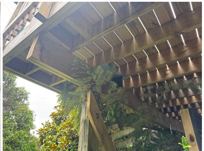
No concerns with the framing structure. Solid and well connected.
