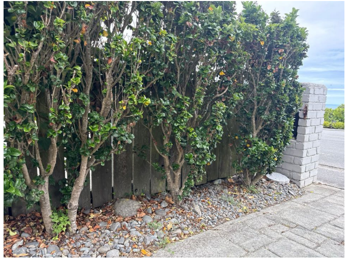
T.H.I.S is unable to comment on the condition of fencing or retaining that are concealed by vegetation.
