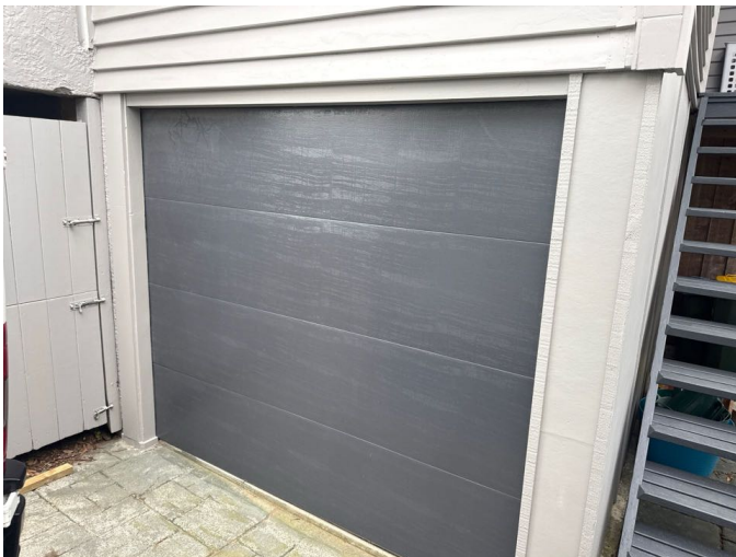
The surface condition of the garage door is good
