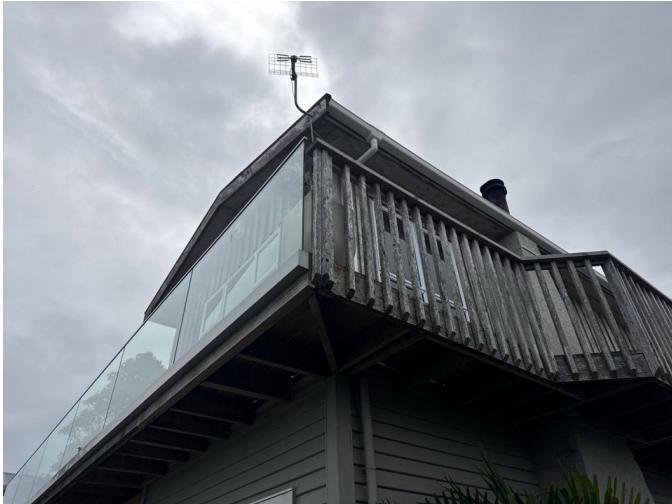
The balustrade is secure
