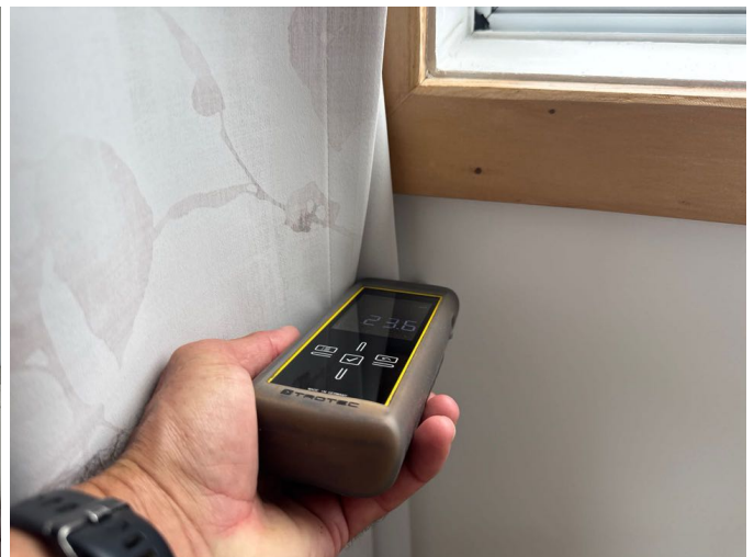
The moisture levels to the external walls were within the normal range
