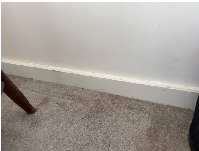
The wall and ceiling linings and carpet are in good condition
