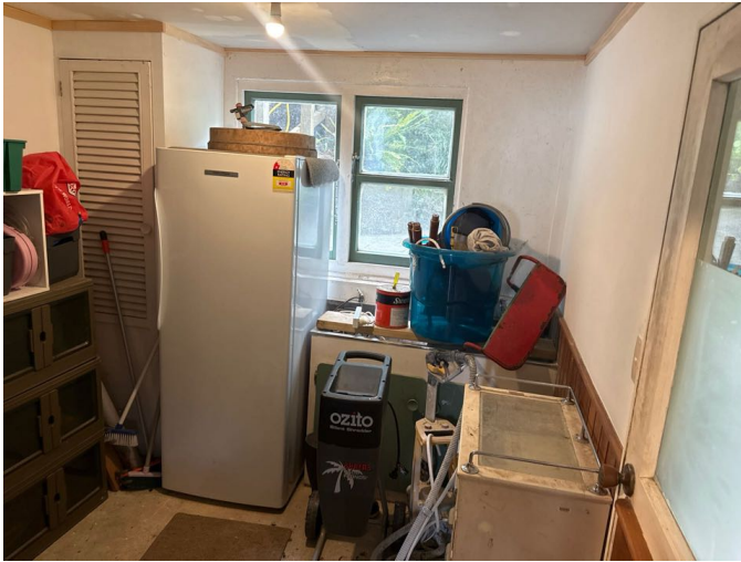
Storerooms to the back of the garage. The tub area was not inspected.
