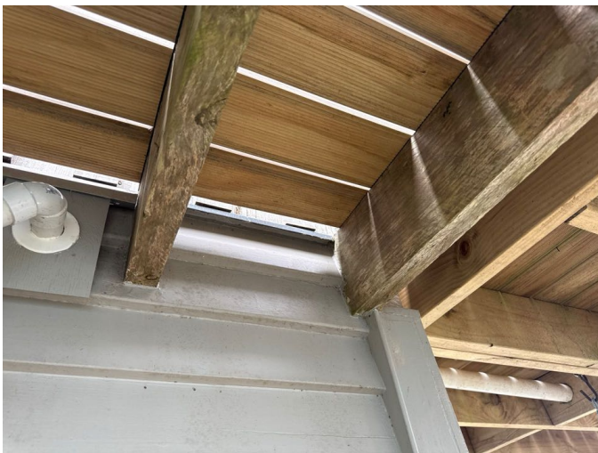
Drainage clearance and flashings installed at the cladding junction.
