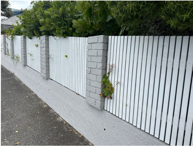
The fencing to the front is intact and solid
