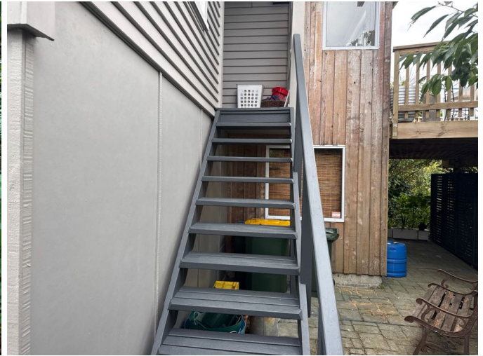
The timber stairs and handrail are solid and secure
