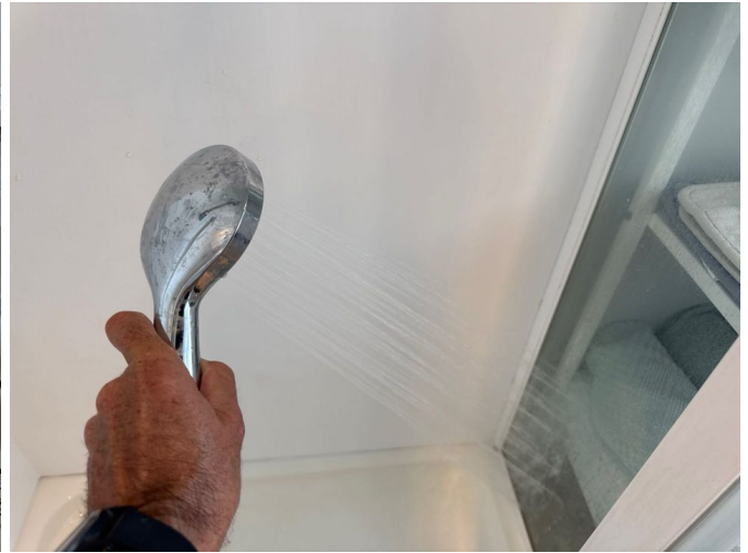
Good water pressure noted. No sign of current leaks from the shower frame during water testing.
