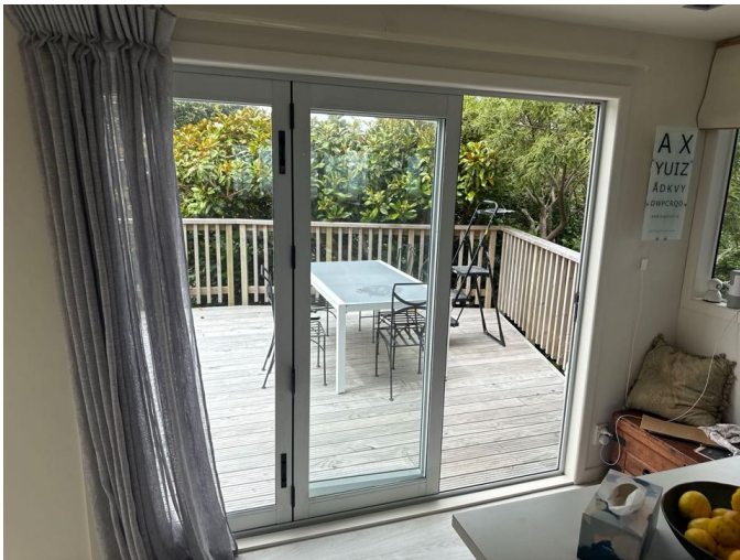
The external doors are functional
