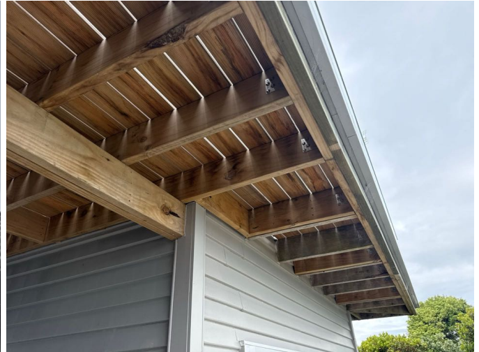
The deck structure has been strengthened and modernised at various locations.
