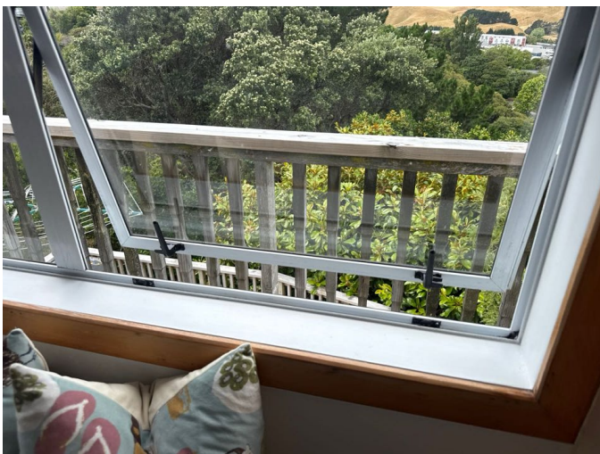
The windows are functioning throughout the home
