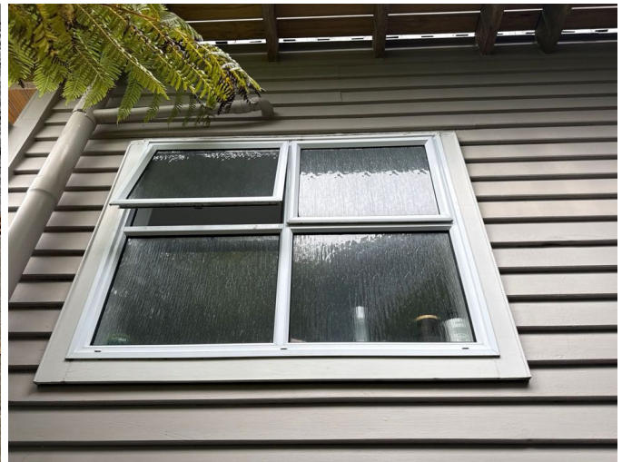
The single glazed aluminium joinery are effectively flashed and sealed
