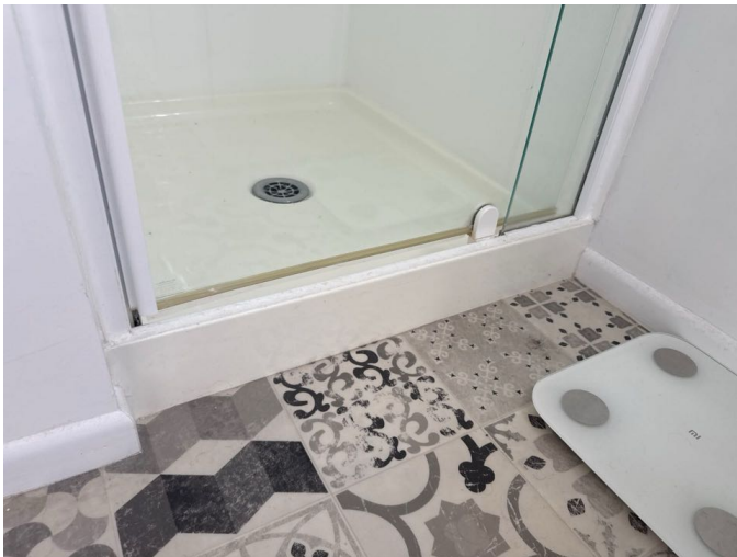
The base of the shower is well sealed
