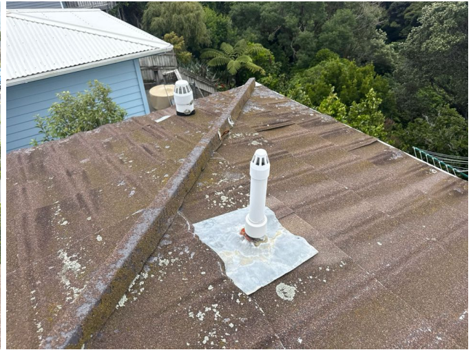
The roof penetrations are effectively sealed
