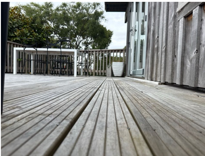
The decking is in good condition
