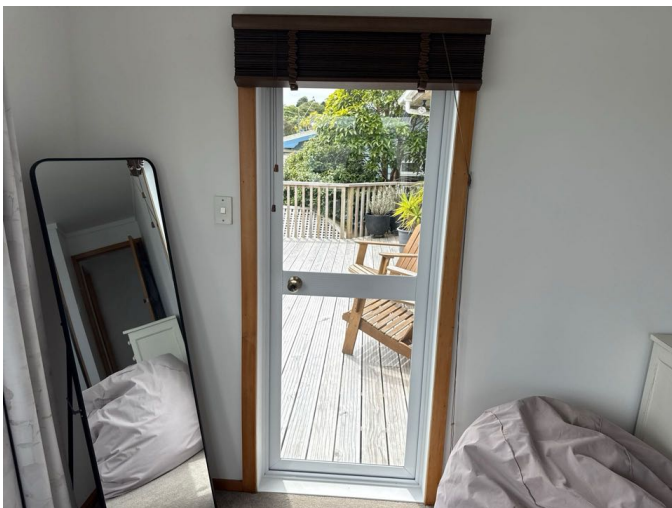
The external door is functional
