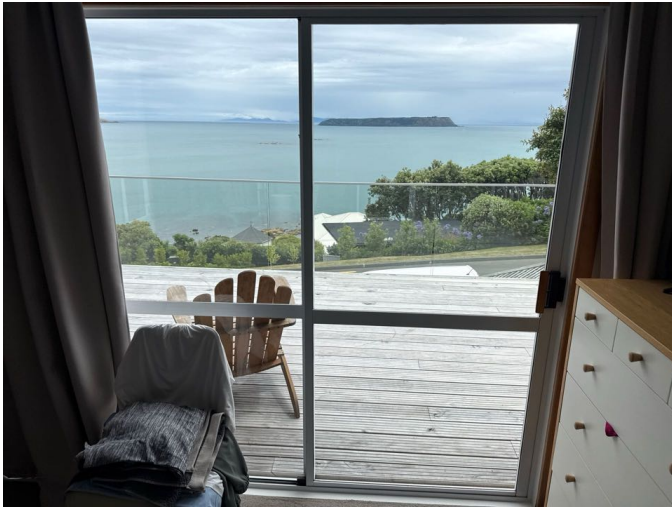
The sliding door is functioning well
