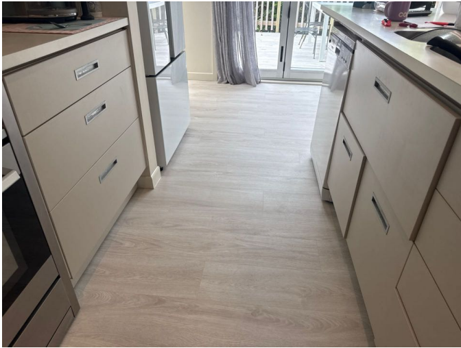
The kitchen cabinetry and vinyl plank floor are in good condition
