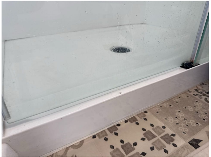
The base of the shower is well sealed. There was no evidence of damage to the shower base at the time of the inspection.
