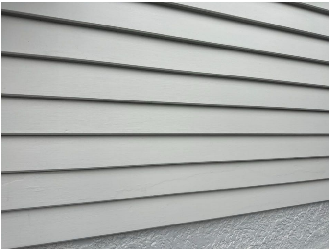
Good paint quality to the timber bevelback weatherboards
